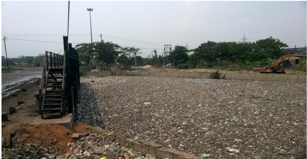
PHOTOS SHOWING THE ACCUMULATION OF FLOATING MATERIALS AT GRATINGS
